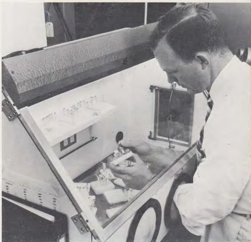
A Bell Telephone Laboratories engineer uses a "dry box" to assemble the new ultra-high-frequency transistor. He is shown placing a metal casing over the transistor to assure long life. Miniaturized electronic equipment is assembled in "dry boxes" to avoid contamination by dirt or moisture. The new transistor can withstand as much as 100 volts over a wide range of frequencies.
