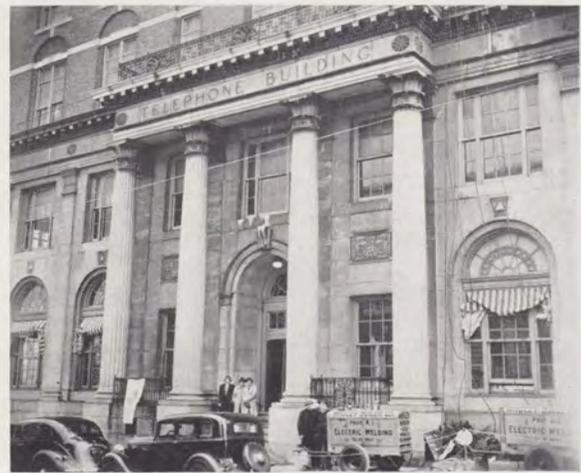
Welding machines provide power for our building, 234 Washington St., Providence, R. I. The flag denotes an emergency red cross station set up within the building.
