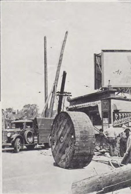
Placing poles at Chicopee Falls, Mass., to support new cables spanning the river after the bridge was destroyed.
