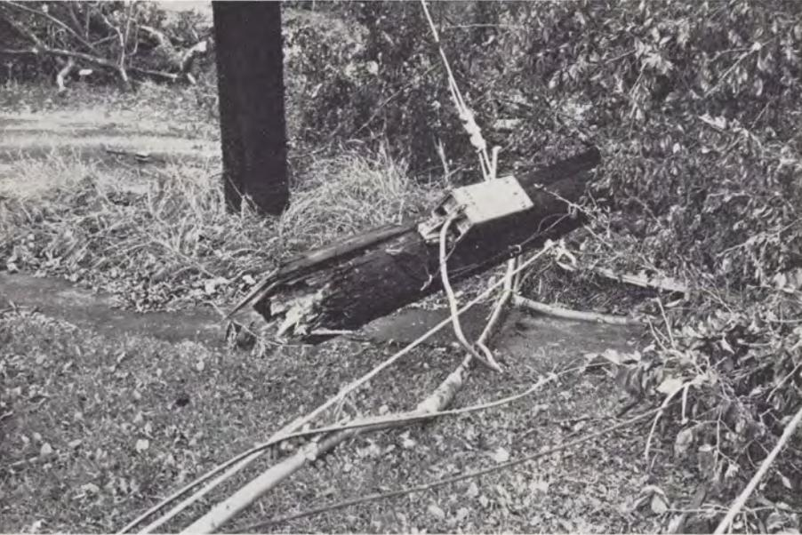
*This pole could not stand the strain, so terminal box, cable junction, guy wire and pole tip crashed among broken branches on Main Street, Brookfield, Mass.*
