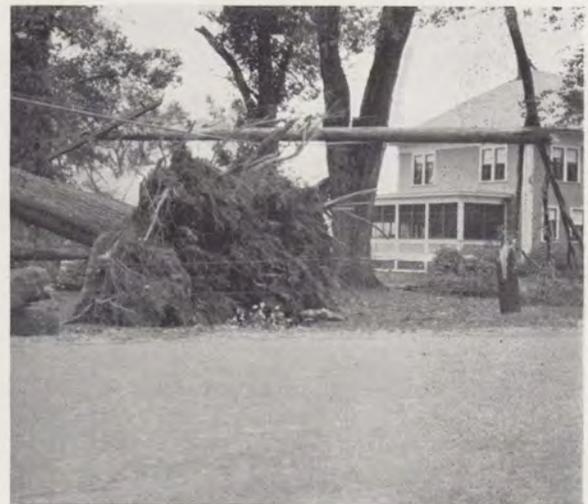
*This cable on Main Street, Northfield, Mass., is suspending a telephone pole in mid-air, leaving only the stump in the ground.*
