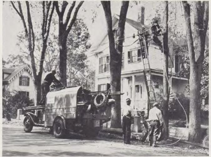
*Truck and crew from the Chesapeake and Potomac Telephone Company repairing damaged wires at Melrose, Mass. The C. & P. was one of the companies which came to our rescue in the storm restoration.*
