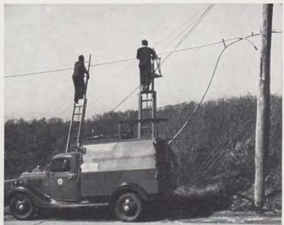
*Cable truck and crew from the Bell Telephone Co. of Pennsylvania repairing broken cable at Narragansett Pier, R. I.*
