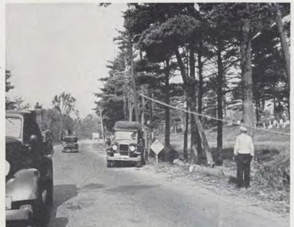
*Truck pulls cable to position on a new pole at Spencer, Mass.*
