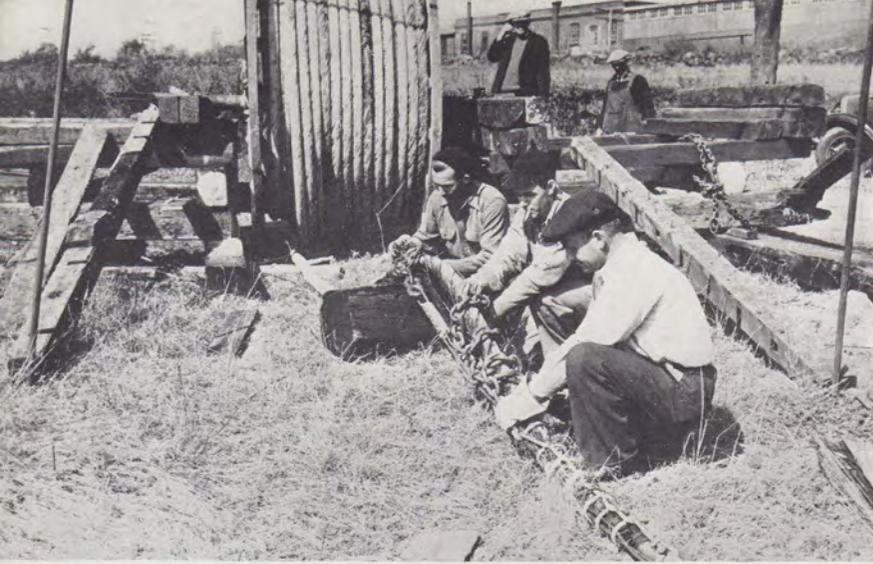
*A step in the process of restoring a submarine cable across the Taunton River, Slades Ferry, Mass. The new cable is prepared for dragging across the bed of the stream.*
