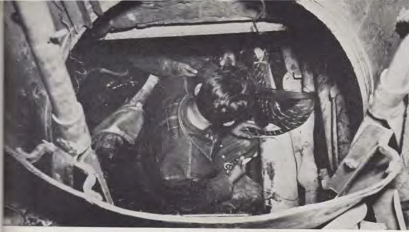
*Splicer at Providence, R. I., who went down into flooded manholes to dry out our cables before the water had been completely pumped out.*
