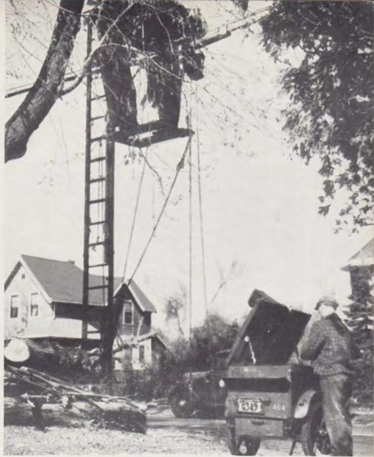
*Cable splicers from the Bell Telephone Company of Pennsylvania working on a 720-pair toll cable in Wakefield, R. I.*
