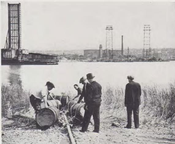
*Another step in the replacement of the submarine cable at Slades Ferry. Steel drums are attached to the cable and winch trucks on the opposite side of the river prepare to drag it across.*
