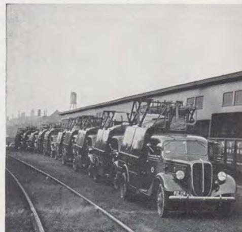
*Some of the 43 pieces of motor equipment loaned by the Illinois Bell Telephone Company to the New England Company for use in reconstructing lines damaged in the hurricane.*
