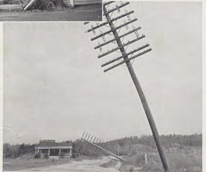
*Shows how the hurricane leveled these sections of open wire toll lines near Southbridge, Mass.*
