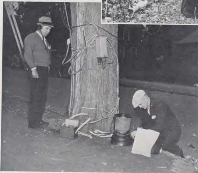
*Using this tree as a telephone pole, these men set up the necessary wires and cable to provide the Melrose Hospital with emergency service after the storm.*
