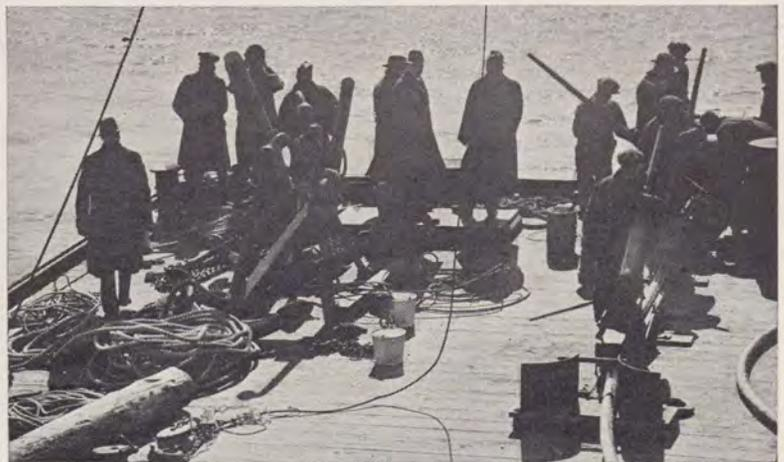
View on the deck of the lighter which was used in the laying of the cable in Mount Hope Bay. At the right may be seen the cable brakes which regulate the paying out of the cable.
