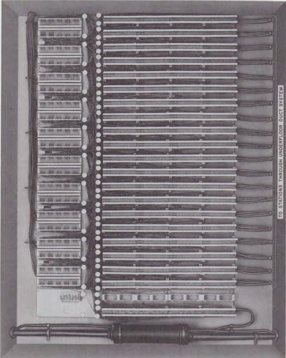
Fig. 16—Typical Apparatus Closet Arrangement Using Modular Apparatus
