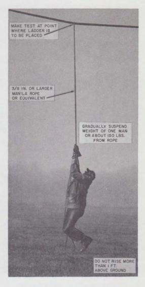
Fig. 2—Testing Strand Prior to Placing Ladder
