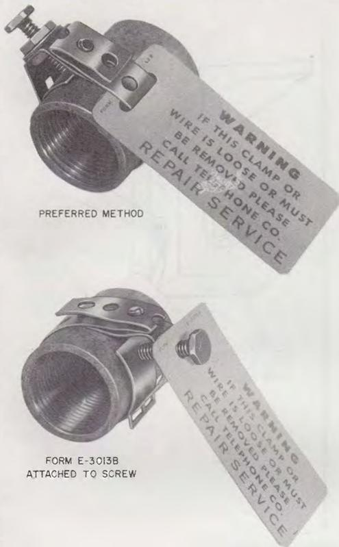
Fig. 54—Form E-3013B Attached to B Station Ground Clamp
